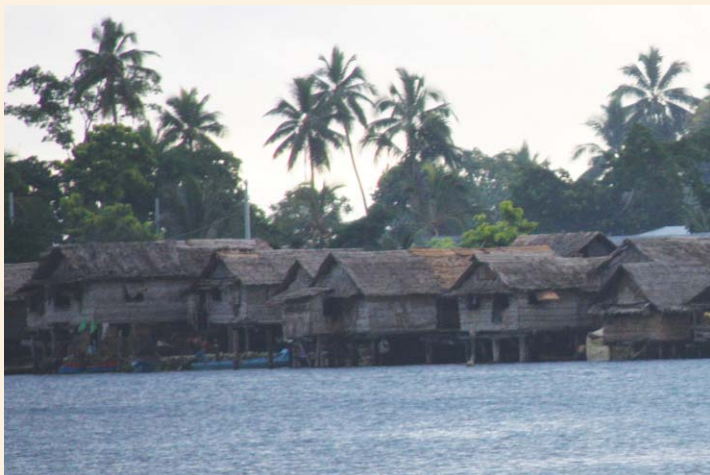
Stilts help protect houses on the Solomon Islands from rising tides.
