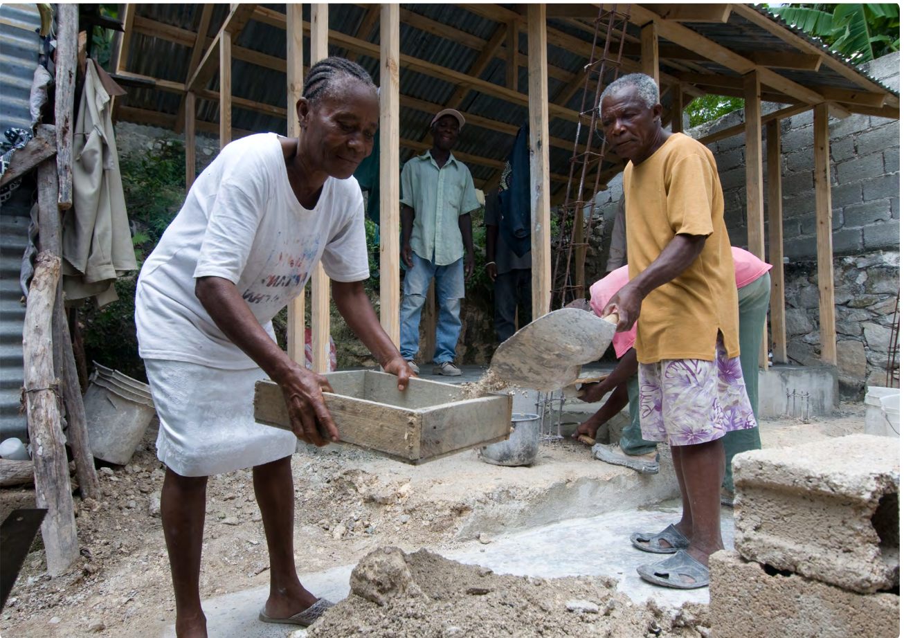
Housing reconstruction in Haiti
